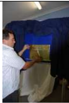
Step 9 Mount Plaque onto Channel and against Backing Panel .- Apply a 100mm strip of self adhesive Velcro Loop tape to the back of your plaque, then apply a 100 mm strip of Velcro Hook tape onto the Loop Tape, Insert Plaque into Channel and attach velcro hook tape to Backing Panel
