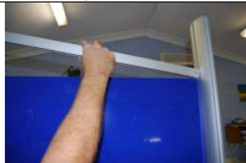
Step 6 Attach upper Rail to posts and align to top of backing panel
