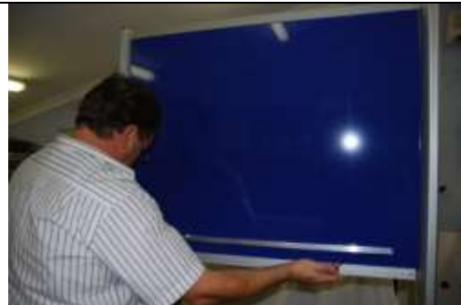
Step 7 Loosen Rail Screws and adjust rails and Backing panel to top of Top Poles, insert caps to top poles, tighten Rail screws
