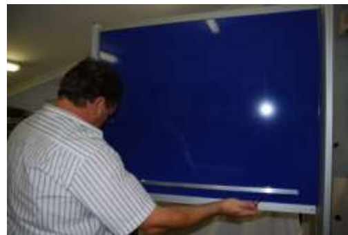
Step 6 Loosen Rail Screws and adjust rails and Backing panel to top of Top Poles, insert caps to top poles, tighten Rail screws
