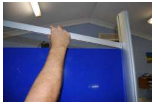
Step 5 Attach upper Rail to posts and align to top of backing panel
